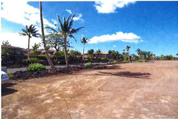
View of a Triangle Lot, camera facing in a southwesterly direction. The Haliu Kai multi-family project can be seen in the background.
