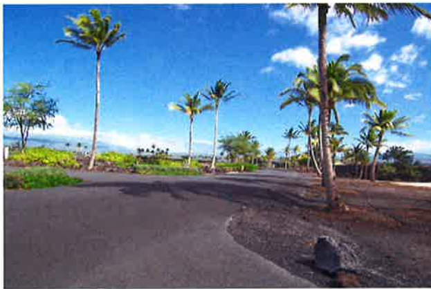
View of the subject roadway exiting the Triangle Lot area. Tier 3 Lots can be seen to the left of photograph.
